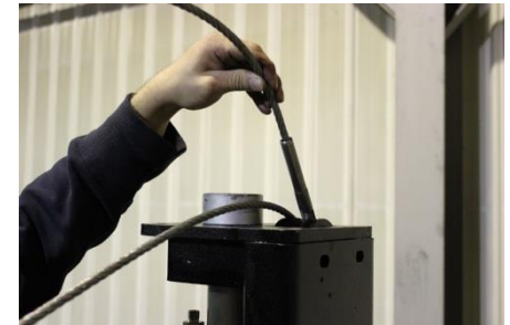
Feed Synchronizing Equalizing Cable into Post 2 BEHIND the existing cable.
